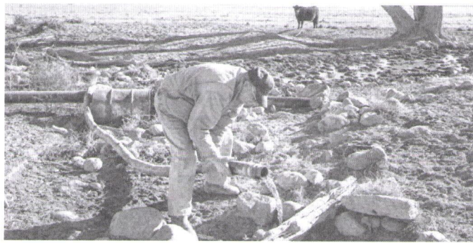
Dean Baker waters his cattle at Baker Rancher on Nov. 20, 2014. Dean was draining the line to keep it from freezing.
