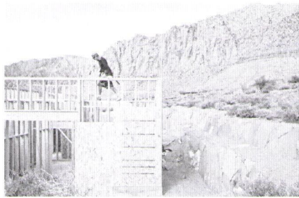
Tony Night works on a home under construction in the Kayenta development on Nov. 19, 2014, in Ivins, Utah.
