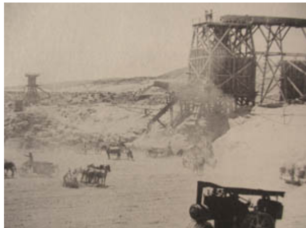
Construction of Lahontan Dam to provide more water for the Truckee Carson project Advertisement
