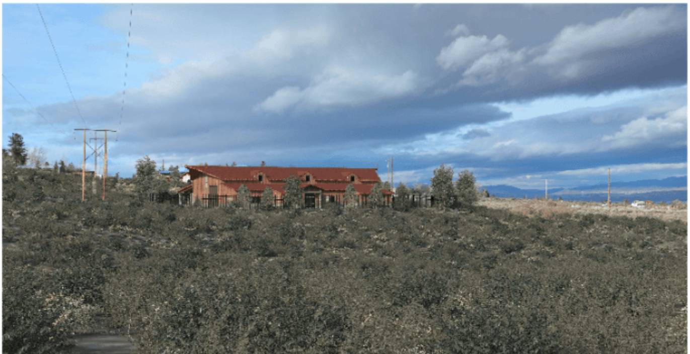
View North of Proposed Water Treatment Plant From Paris Ct/Callahan Ranch
