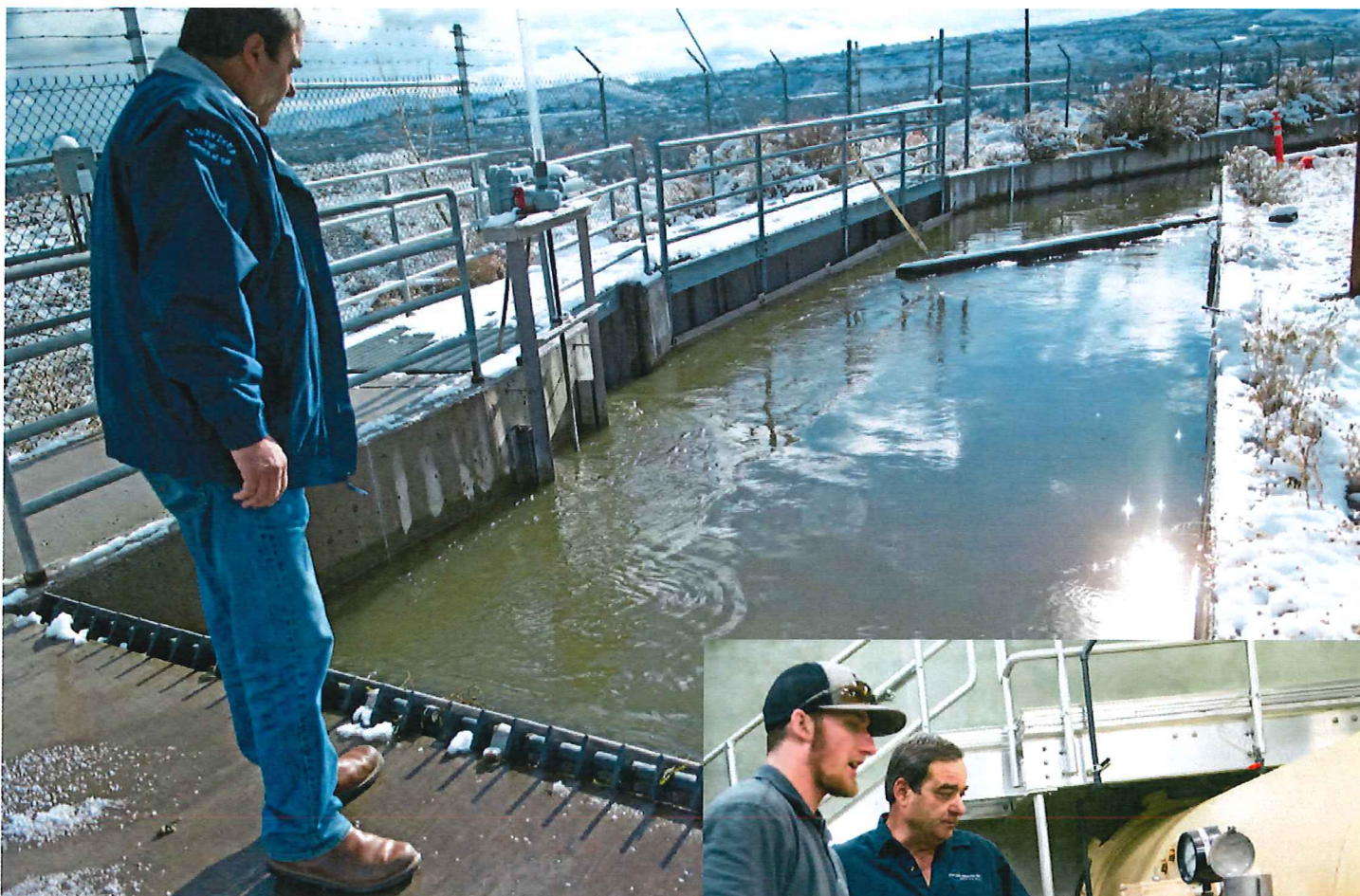
ABOVE: Scott Knecht checks bar screens where raw water is delivered. RIGHT: Knecht discusses the rapid mixer and jet diffuser with Dillon Hansen, apprentice operator.
