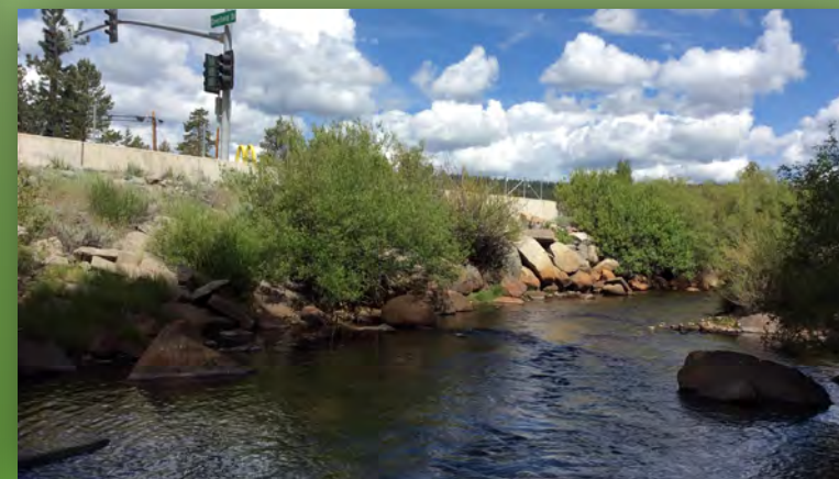
Heavily armored bank immediately upstream of the project site. Photo by Jai Singh, cbec (2015).
