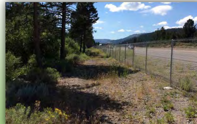
Existing buffer between I-80 (right) and Donner Creek (left). Photo by Jai Singh, cbec (2015).
