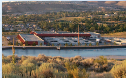
Chalk Bluff Water Treatment Plant
